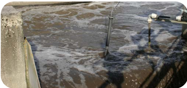
In the aeration basin: calibration free FDO® 700 IQ for dissolved oxygen
