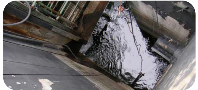
In the aeration basin of a WWTP with industrial wastewater: ViSolid® 700 IQ Suspended solids sensor with ultrasonic cleaning
