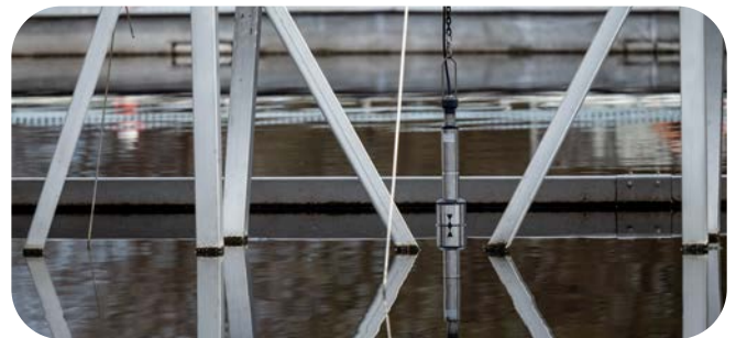
In the post-sedimentation: IFL 700 IQ Ultrasonic sensor for detailed presentation of sludge profile
